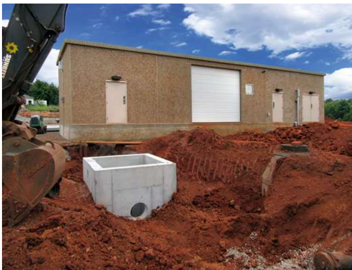
20 ft by 60 ft by 12 ft Easi-Span building.
