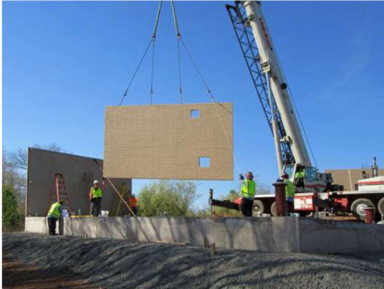
Panel erection using crane.
